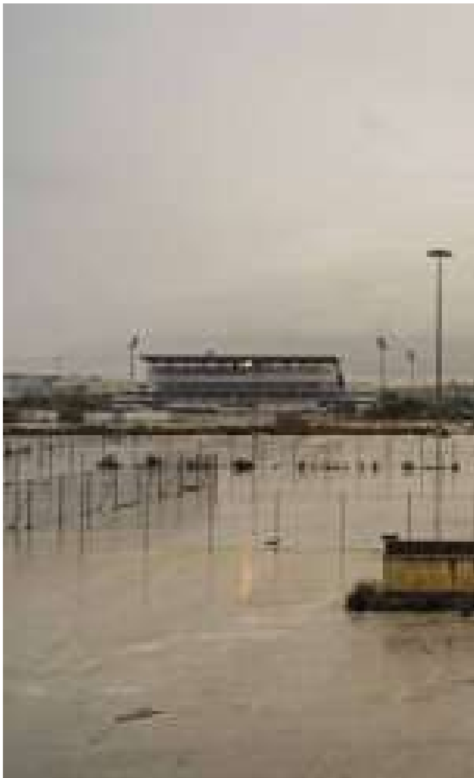
Partial view of the West Airport, 2020.
