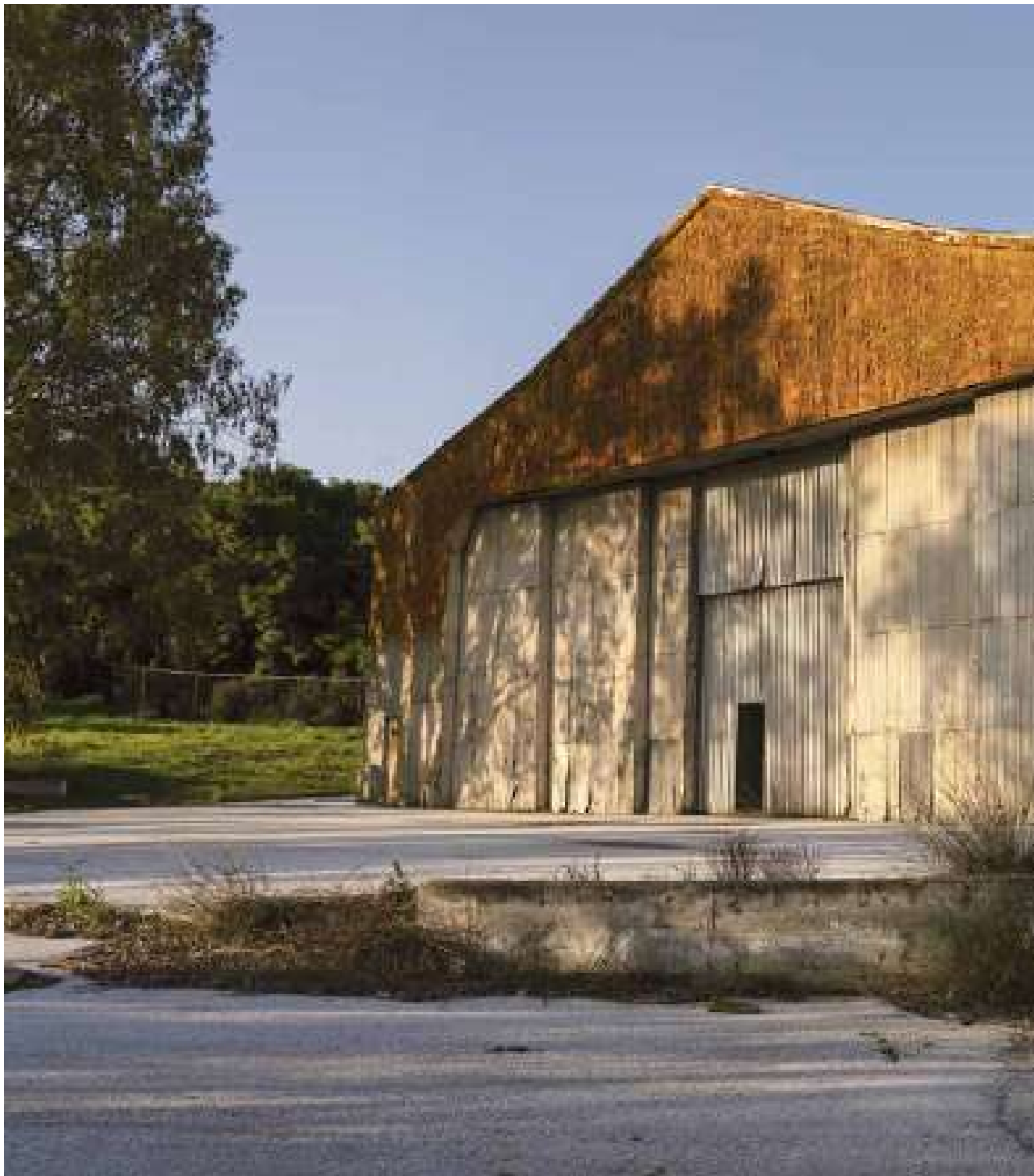
The British Hangar, known as the 'Pagoda', which was constructed by the British in the years 1940-1941 and was used initially as a warehouse, 2020.
