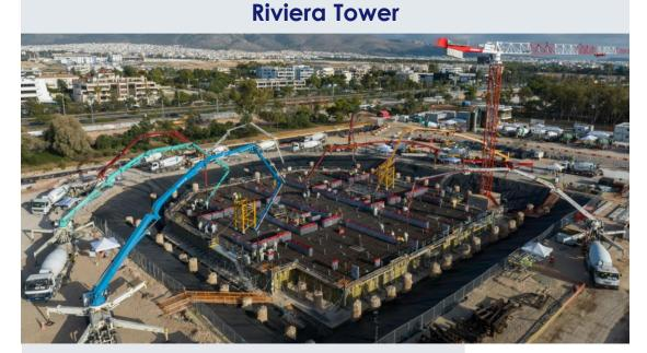
Piling (316 piles, up to 55m depth)Diaphragm Wall (520m, up to 15m depth)Tower excavation works & dewateringConcreting of the Tower foundation slabConcreting works for Podium (2 levels)Concreting works for Tower lobby floor slabConstruction milestone (Tower lobby casting)
