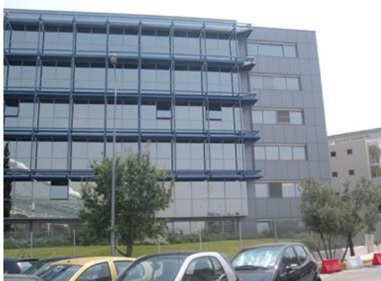
External View of the building
