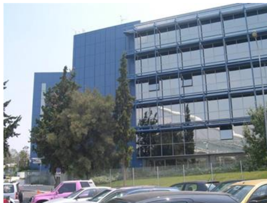
External View of the building
