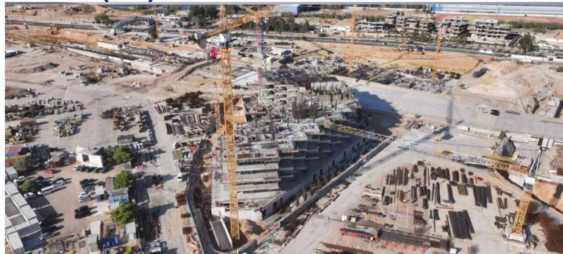
4 th floor concreting works in progress
