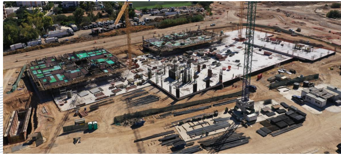
Concreting works in progress
