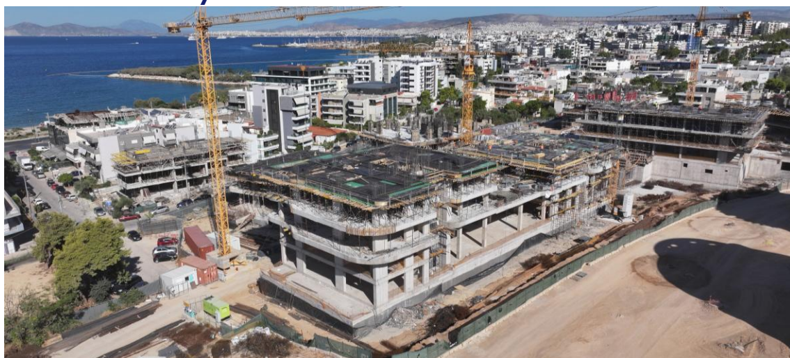
Superstructure concreting works in progress
