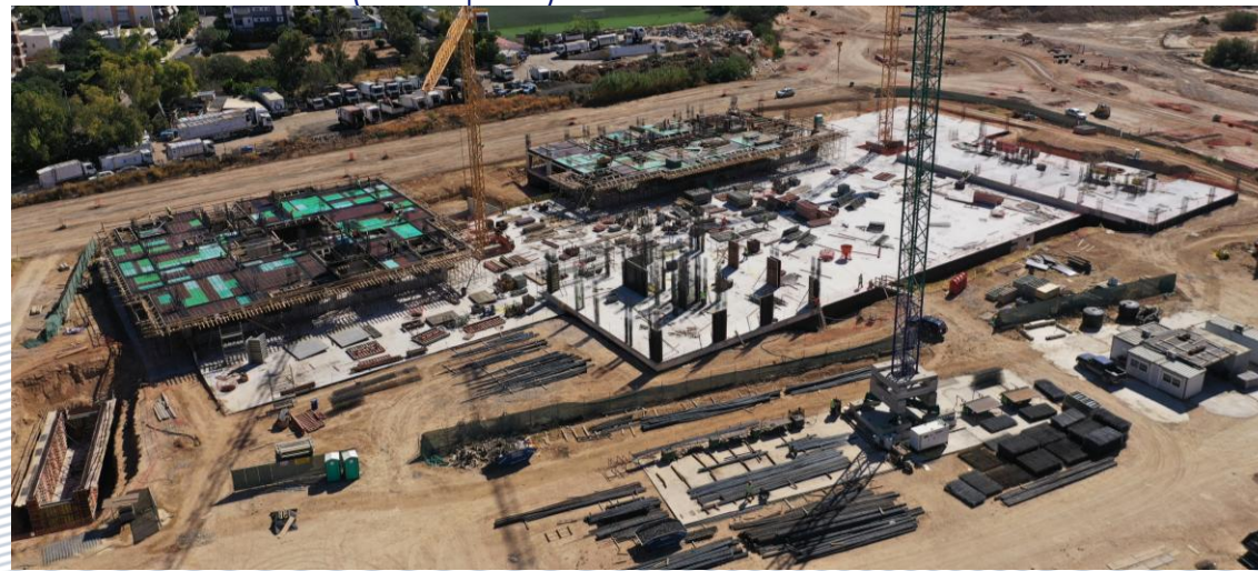
Concreting works in progress
