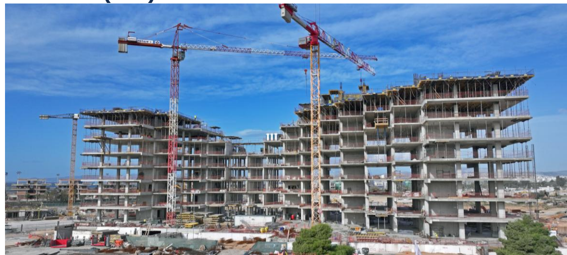
6-7 th floor concreting works in progress
