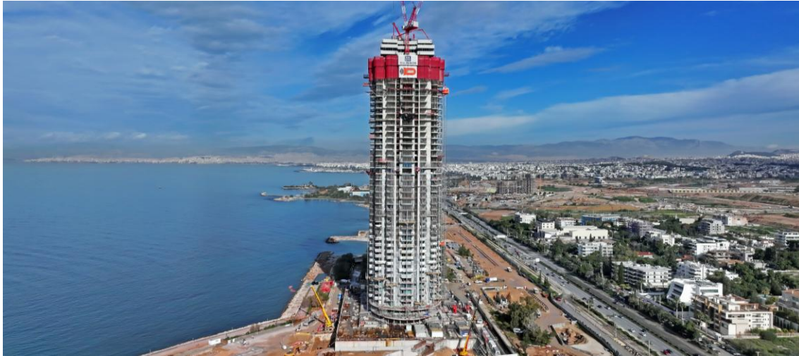
Concreting works: 48 th level Core Structures & 46 th level Slabs
