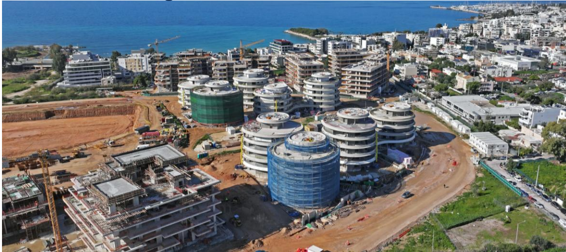
Plots 6.9-6.10: Main works in progress
