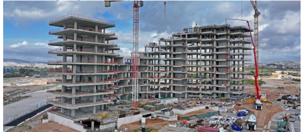
Superstructure concreting works completed. Main works in progress.
