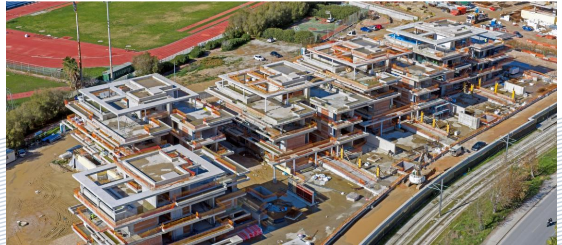
Plots 7-8 : Main works in progress
