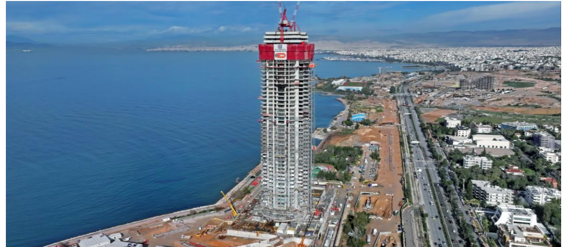
Concreting works: 48 th level Core Structures & 46 th level Slabs
