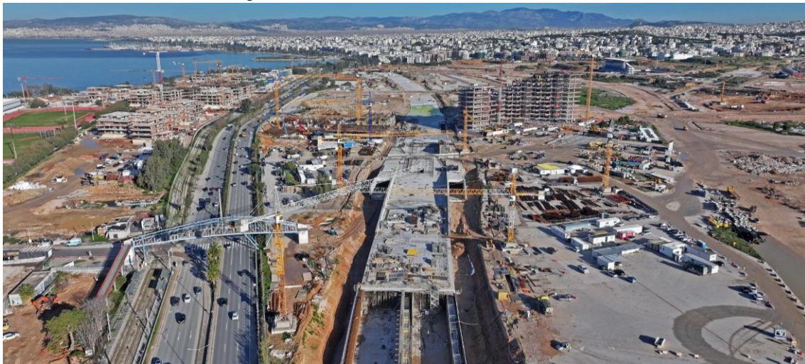
96% of excavations & concrete casting completed to date
