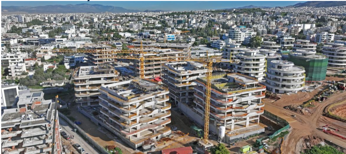
Superstructure concreting works completed. Main works in progress.
