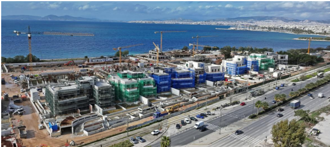
Plots 5-6 : Main works in progress
