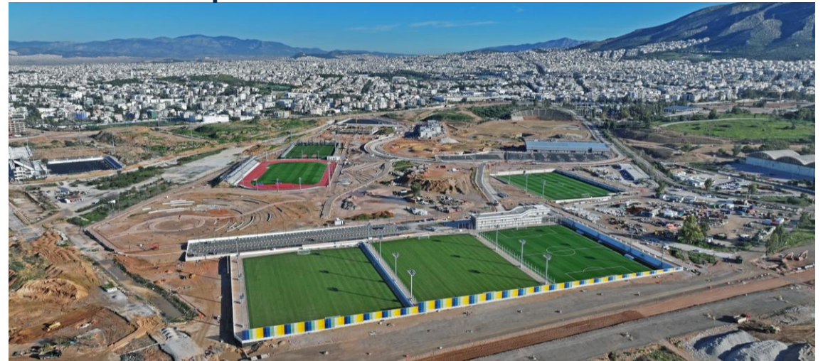
Track and field & throwing field, football pitches & admin build. completed
