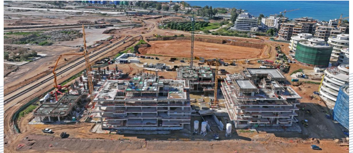
Concreting works in progress in Plot 6.7 . Excavations completed at Plot 6.8
