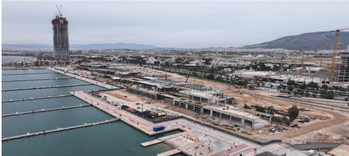
99% of concreting works completed to date. Fitout works in progress.
